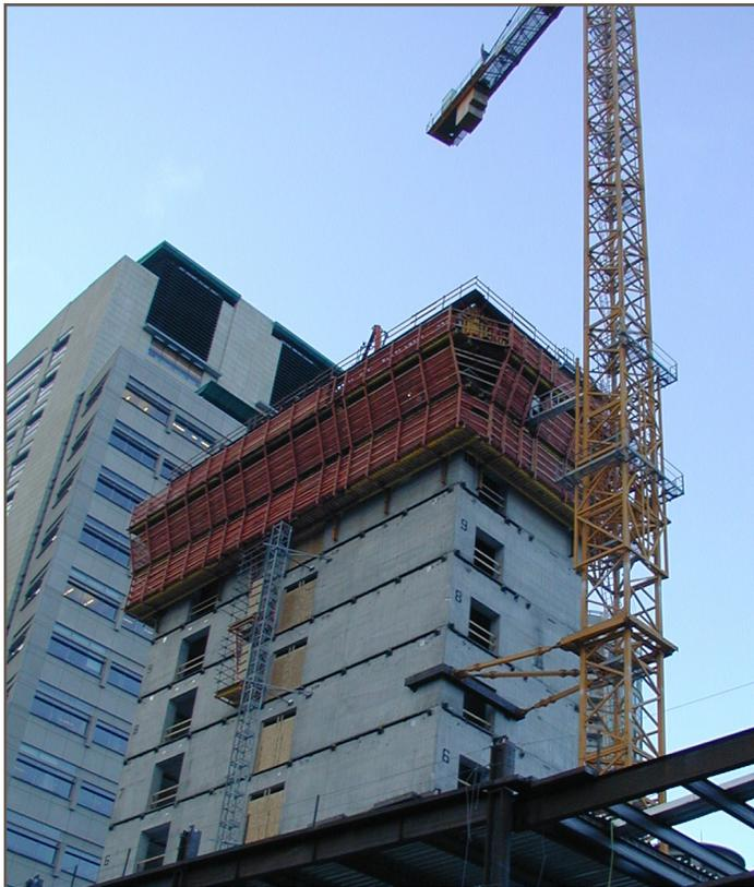
*At West 8th, core construction set a record for cycle time for its type of Peri system, often just three days per cycle on floors 14-28.*
